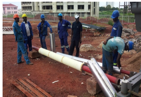
ON-FILED PIPE FOAMING
